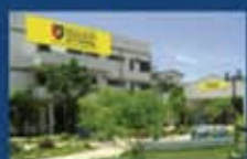
CAMPUS LAURO DE FREITAS
